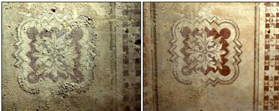
Santa Maria Novella Basilica in Florence, wall paintings by Andrea da Firenze: conservation carried out by means of lime/alcohol dispersions
